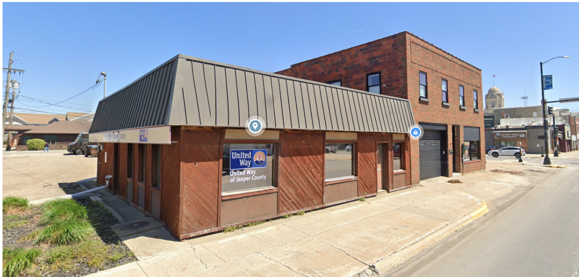
Existing Conditions Photo, courtesy Google Street View
