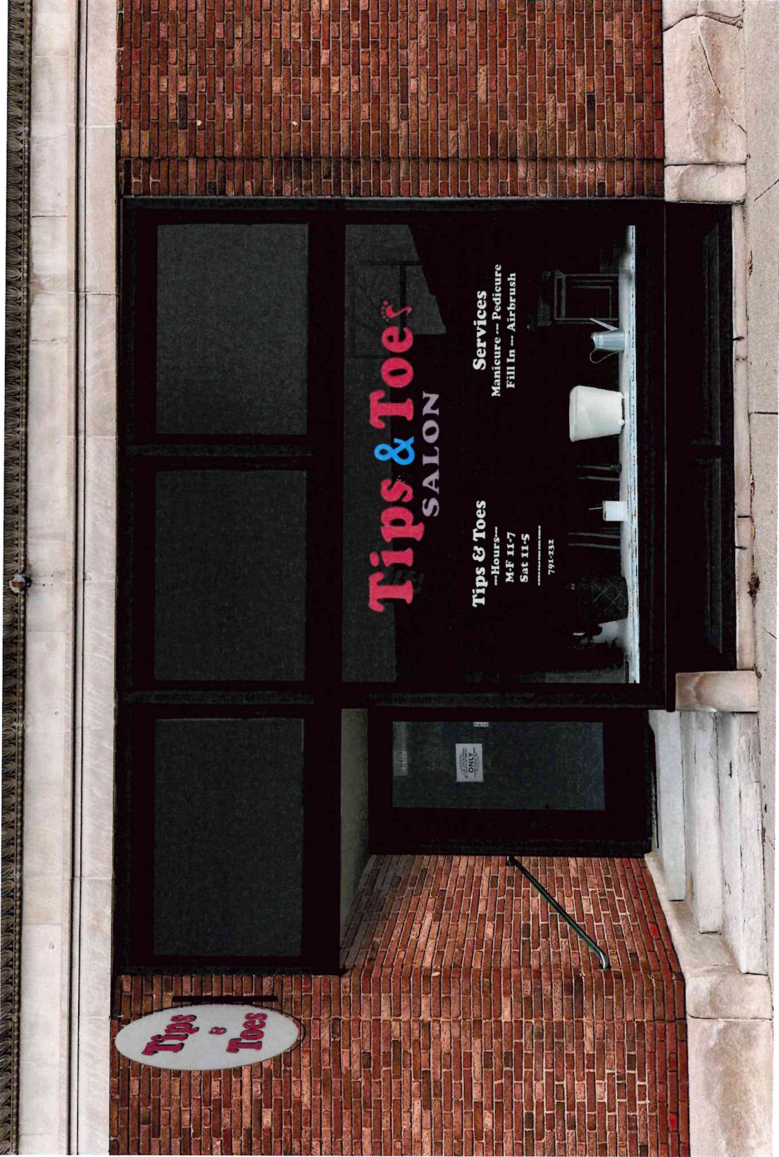
Design option showing transom windows with single display window, and projecting signage.
