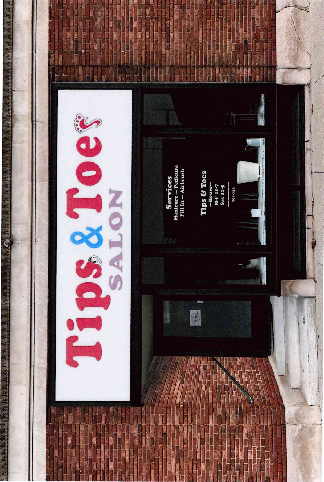
Design option showing sign band in the transom and three-part display window.
