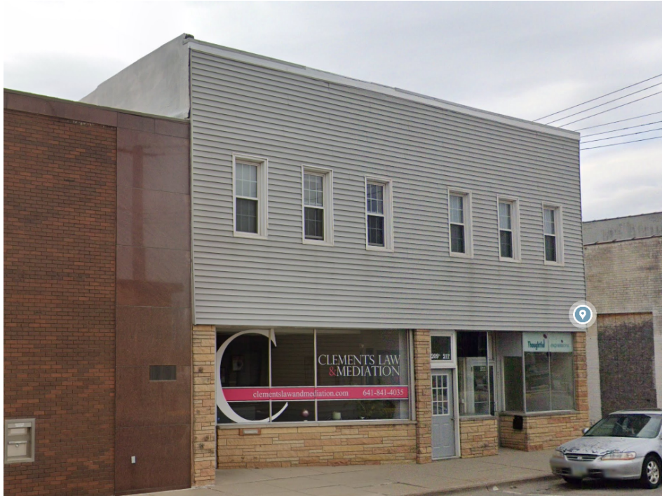
Existing Conditions Photo, courtesy Google Street View
