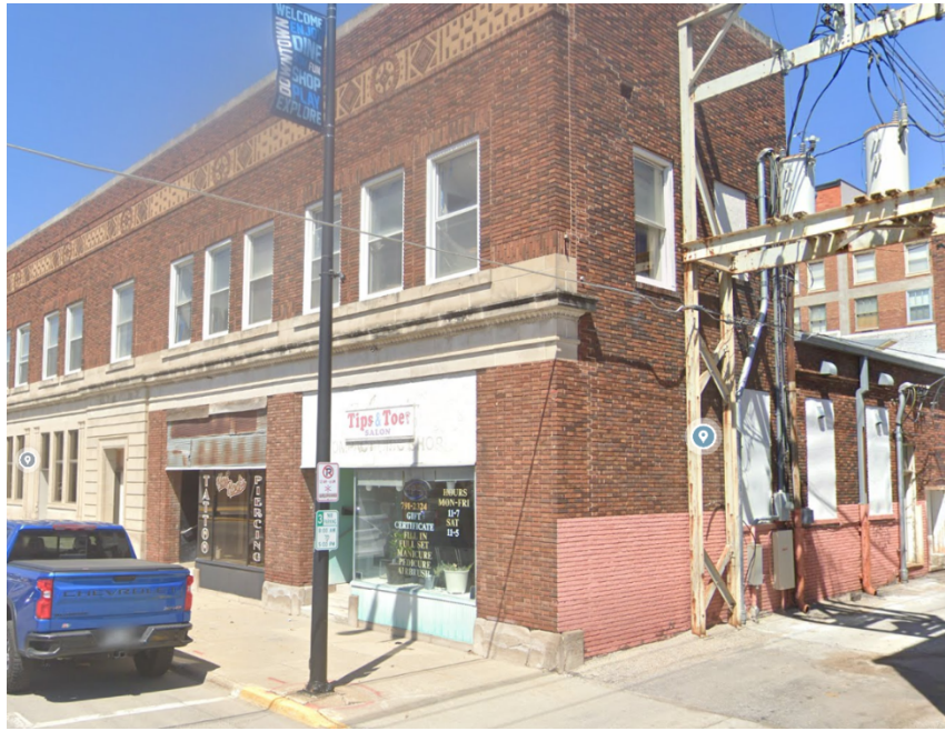
Existing Conditions Photo, courtesy Google Street View
