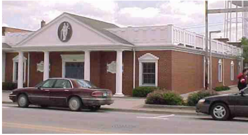
2023 Photo of the front Subject Building
