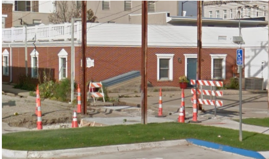
2023 Photo of the rear of Subject Building
