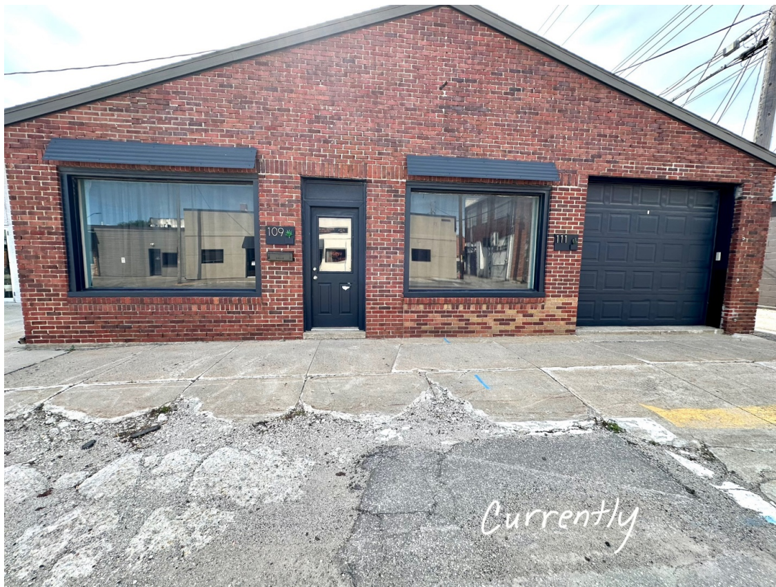
Building Façade off of W 3 rd St. N
