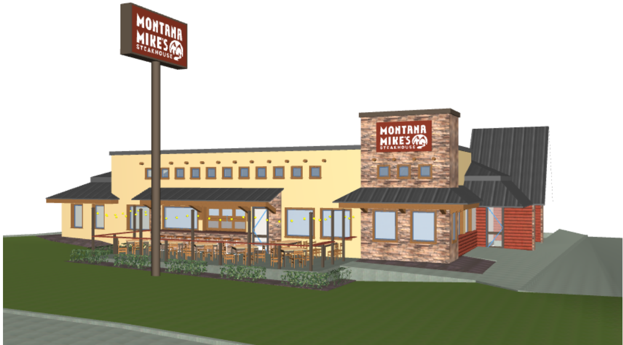
Figure 5: View from the street
