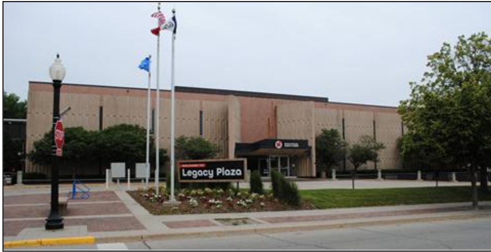
Figure 18. East façade of Building 20, looking west. Tallgrass Archaeology LLC photograph, 6/8/2025.
