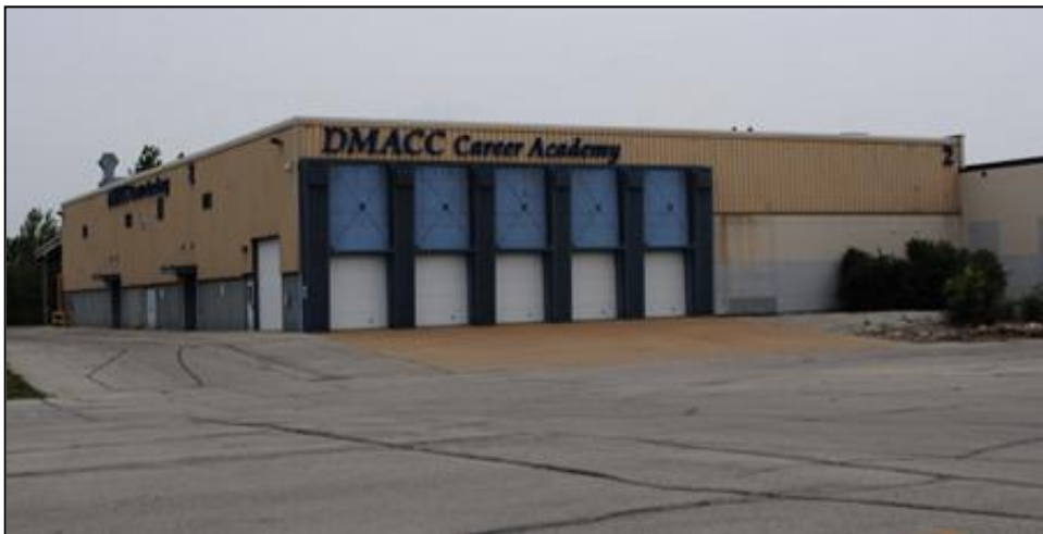
Figure 27. The south and west sides of Building 86, looking north-northeast. Part of the adjoining Building 36 can be seen at the far right of the photograph. Tallgrass Archaeology LLC photograph, 6/8/2025.
