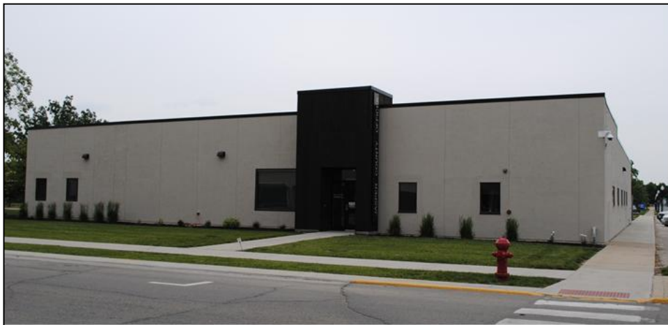
Figure 26. Building 83, currently a Jasper County-owned office building, looking east. Tallgrass Archaeology LLC photograph, 6/8/2025.
