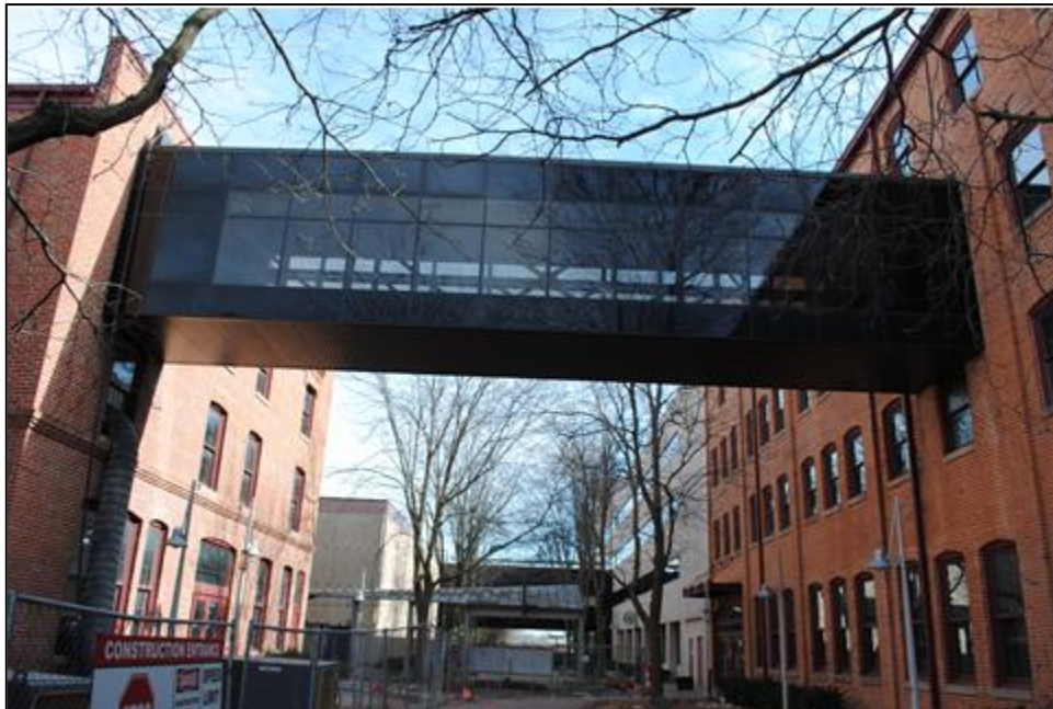
Figure 21. West side of Skywalk/Building 34 connects Buildings 1 and 16; Building 98, visible in the background, connects Buildings 17 and 20, looking east. Tallgrass Archaeology LLC photograph, 2/28/2025.
