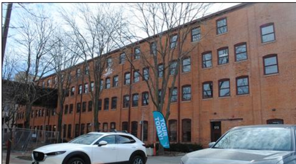
Figure 11. South wall of Building 16, looking southeast. Tallgrass Archaeology LLC photograph, 2/28/2025.
