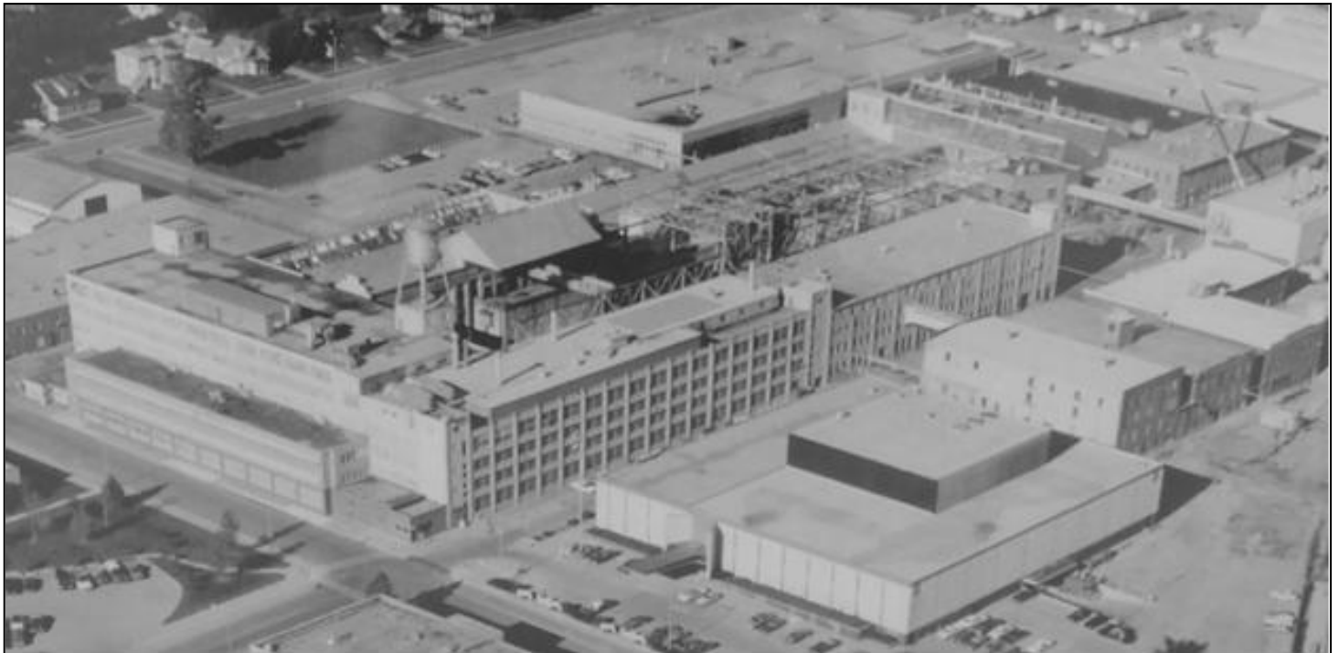
Figure 69. Aerial photograph of the Maytag Plant No. 1 circa 1986, looking southwest, not long before the major modification of Buildings 17 and 18. Note the additions on the east side of Building 18 that have also been removed. Source: Newton Enterprises LLC 2014:113.
