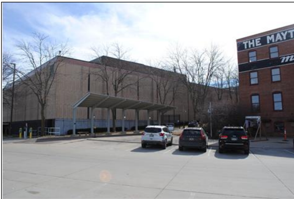
Figure 28. Plaza landscape situated between Building 1 (right) and Building 20 (left), looking southeast. The metal canopy near the center of the photograph is one of two, both extant, added in or shortly after 1988. Tallgrass Archaeology LLC photograph, 2/28/2025.
