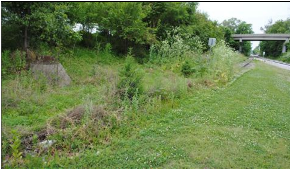
Figure 32. View of the only railroad spur track left within the district, looking west. This track runs from the current Iowa Interstate Railroad Tracks (right) into the district, and to a railroad bumping post (not visible). All other tracks from the extensive rail yard/sidings/spurs in the district have been removed. Tallgrass Archaeology LLC photograph, 6/8/2025.
