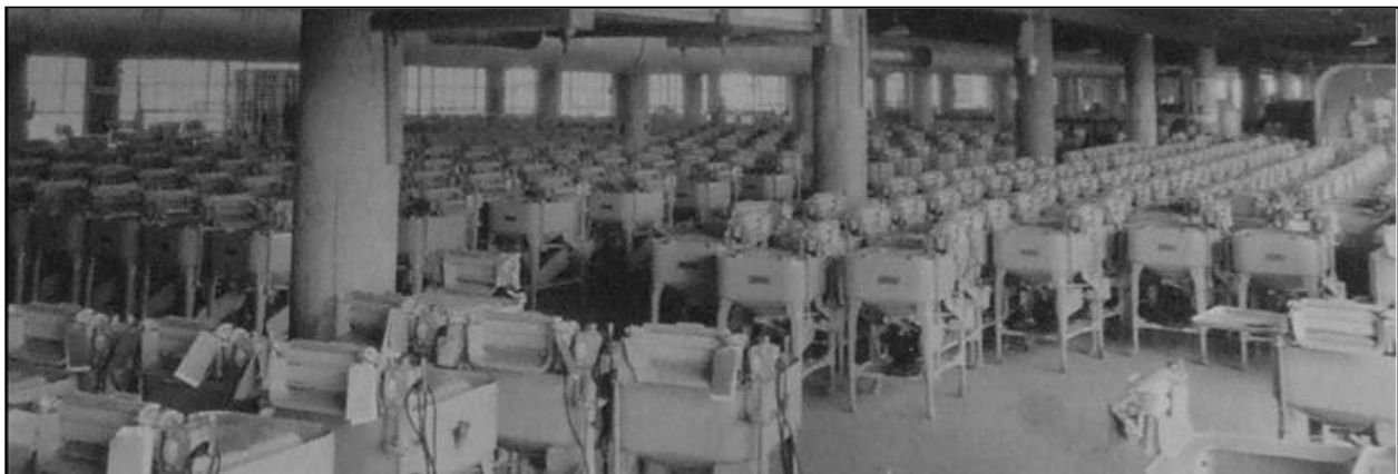
Figure 45. Interior view of Building 17, with a large number of finished Gyrafoam units ready for shipment, unknown year. Note the columns. Source: Newton Enterprises LLC 2014.
