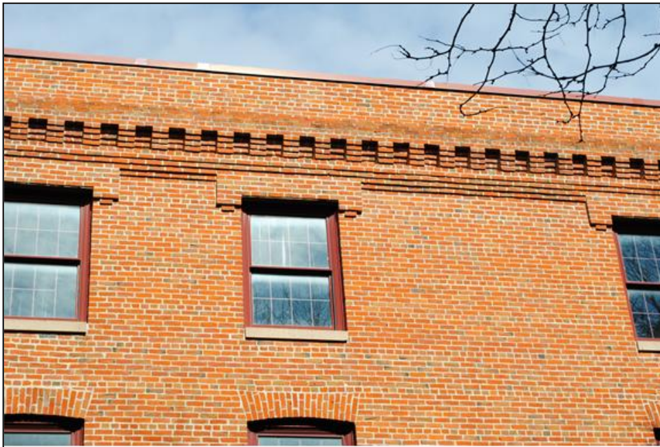
Figure 5. Detail view of masonry on Building 1: cornice and fenestration details on the east part of Building 1's south wall, looking north. Tallgrass Archaeology LLC photograph, 2/28/2025.
