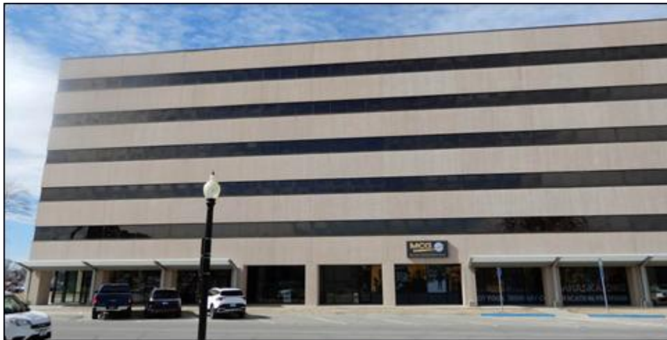
Figure 15. East wall of Building 18, looking west. Tallgrass Archaeology LLC photograph, 2/28/2025.
