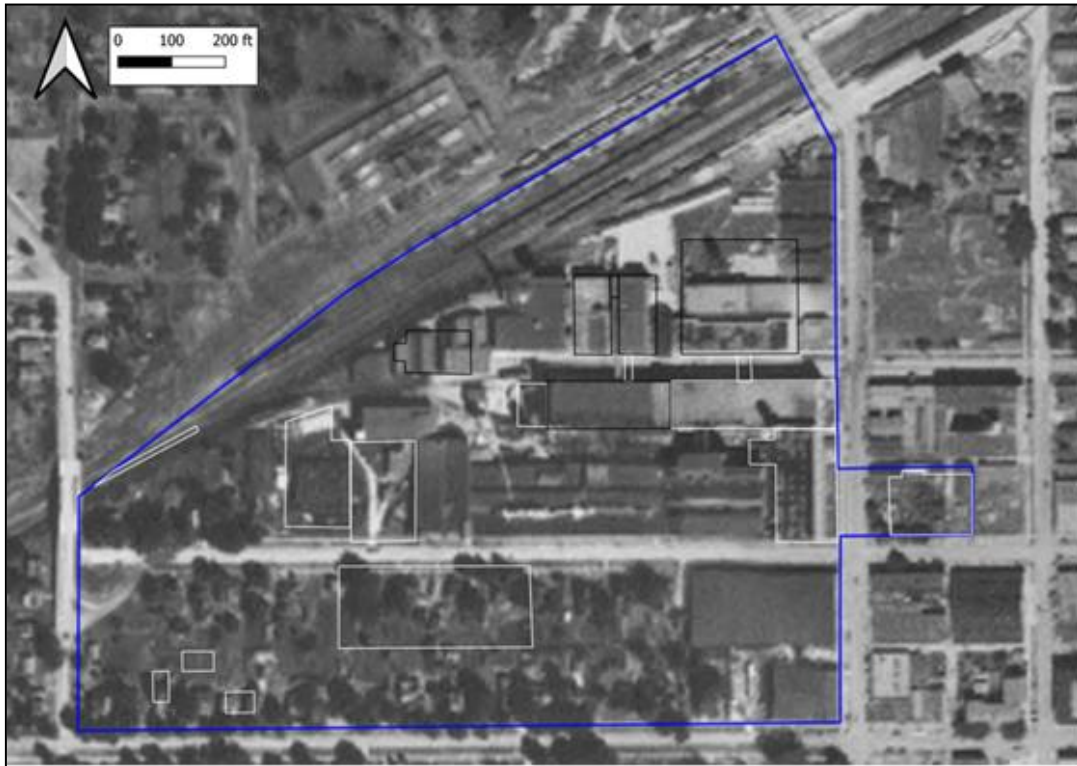
1930s historic aerial image of Newton, showing the district boundary (blue), contributing resources (black) and non-contributing resources (white).
