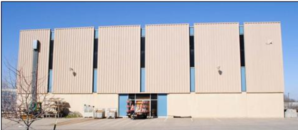
Figure 25. South wall of Building 82, looking north. Tallgrass Archaeology LLC photograph, 2/28/2025.
