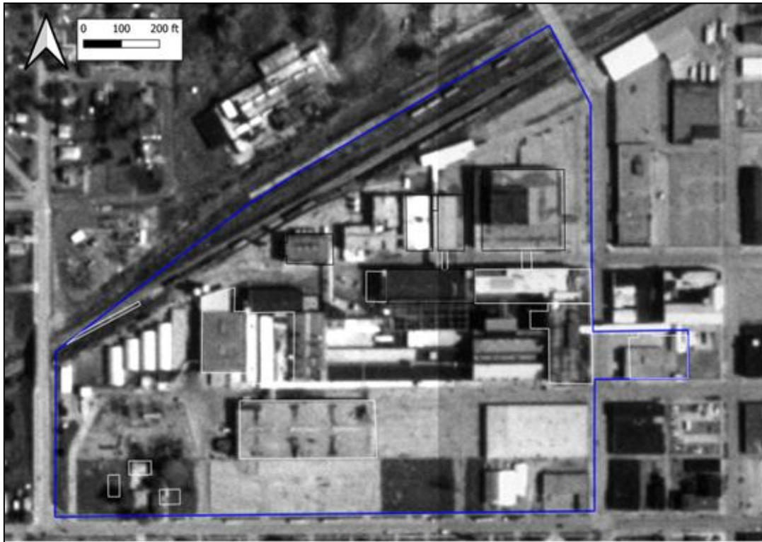
1980s historic aerial image of Newton, showing the district boundary (blue), contributing resources (black) and non-contributing resources (white).
