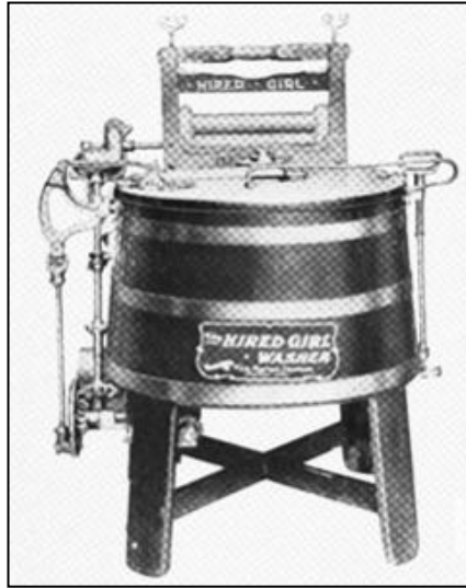
Figure 42. Image of a “Hired Girl” belt driven washing machine, 1909 (Image Source: Maytag Company 1945:13).
