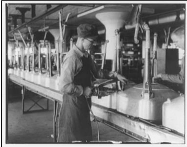
Figure 46. Attaching Legs, Building 18 (Theodor Horydczak Collection, Library of Congress). Note the mushroom columns in the rear of the photograph.
