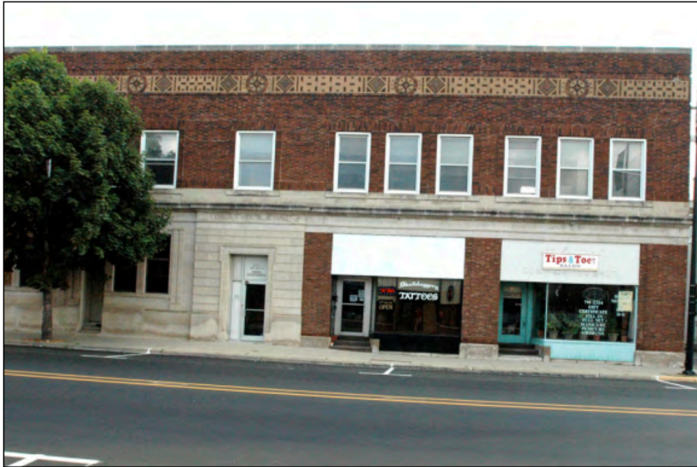
View of the south elevation of the Jewel Building looking north across 1 st Ave. E. The entrance to the upstairs apartments is numbered 104, and the two bays (from left to right) carry the numbers 108 and 110 1 st Ave. E.
