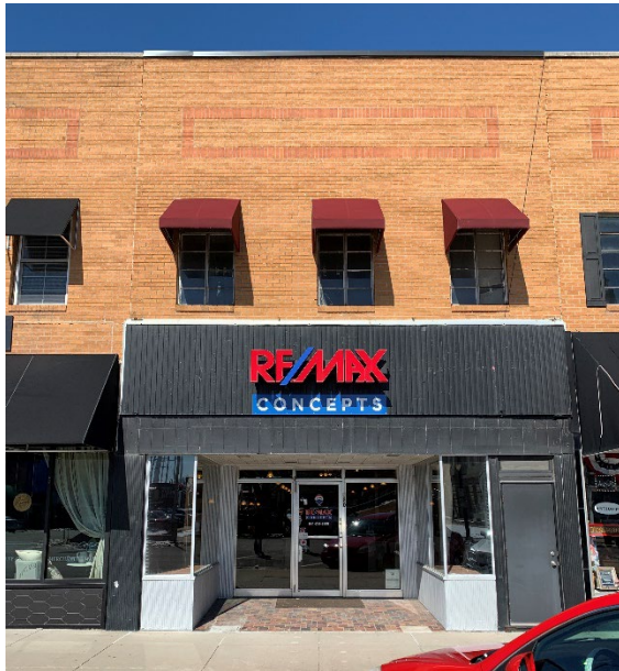
Existing Front of Building
