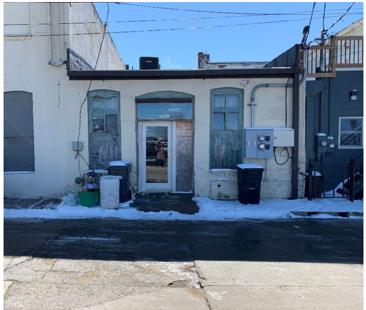
Existing Back of Building
